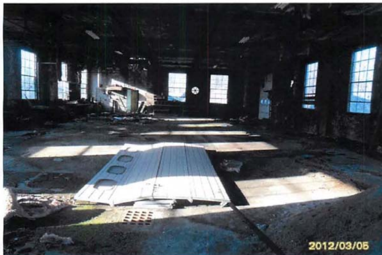
Interior of former Highway Garage, looking from front to rear.
